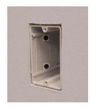
4. SliderBOX<sup>TM</sup> will be mounted flush with drywall at this point.
