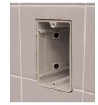
5. Re-tighten the slider plate mounting screws.
