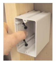
1. Position slider plate forward so box will mount in its normal position for nominal drywall thickness.
