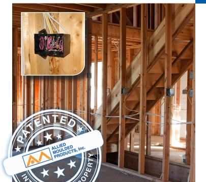
United States Patent 6,365,831 B1 covers the topic of electrical boxes which include clamping devices used for securing electrical cable to the electrical box in accordance with the National Electrical Code, Section 370-17(c).
