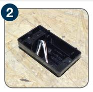
Move floor box in highest position by loosening slider plate screws, install sub floor around raised box
