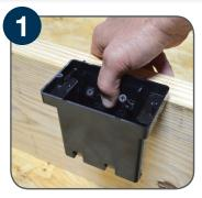
\*Find and install floor box on solid floor joist; mount with slider plate in the "up" position
