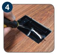
Adjust box height to achieve a flush position; wire the included device and install the gasket and cover
