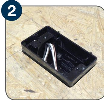
2 Move floor box in highest position by loosening slider plate screws, install sub floor around raised box
