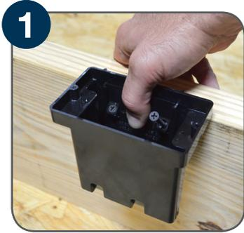
1 \*Find and install floor box on solid floor joist; mount with slider plate in the “up” position
