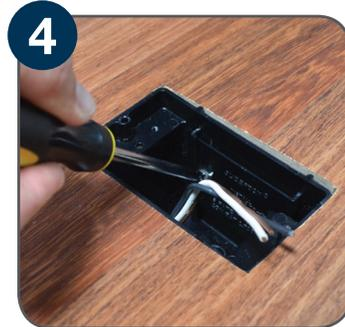
4 Adjust box height to achieve a flush position; wire the included device and install the gasket and cover
